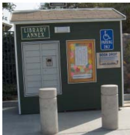
The library annex's location provides round-the-clock access for library patrons.
